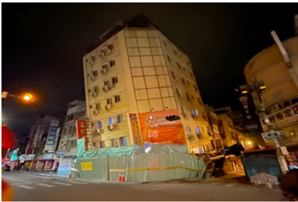
The Full Hotel building in Hualien, which had been previously damaged in the 3 April Taiwan earthquake, tilts further after a series of earthquakes on April 22-23. Image Source: CNA/AFP
