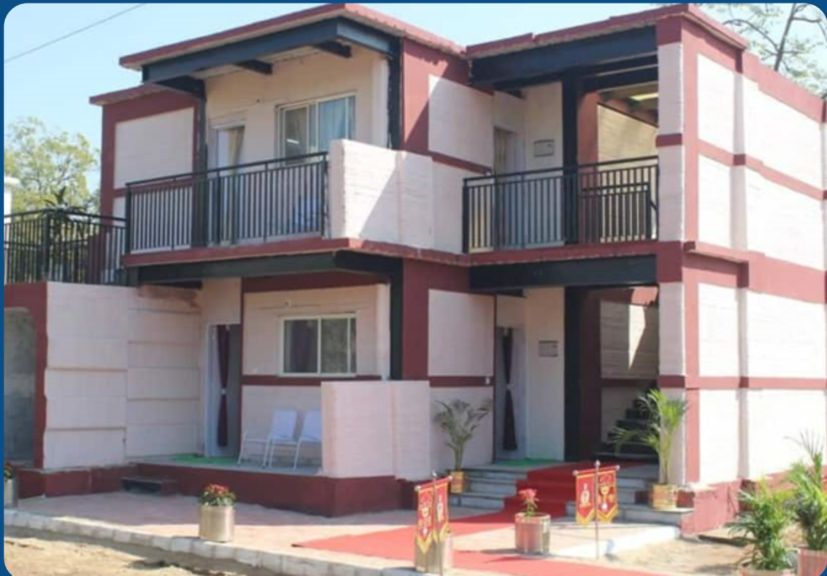
Figure 2: Construction work of the dwelling unit measuring 71 sqm with garage space was completed in just 12 weeks by utilising the 3D printed foundation, walls and slabs | Source: Financial Express
